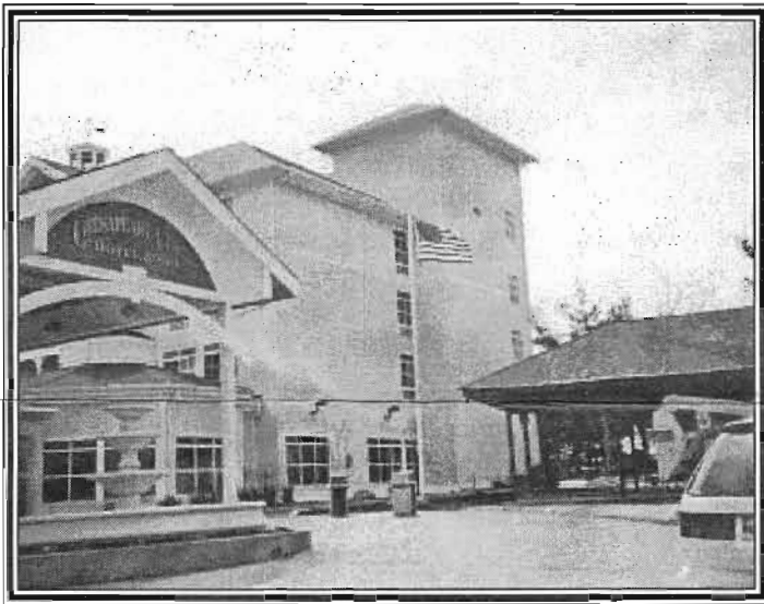
Front view of the new Chesapeake Beach Hotel & Spa. Photo by Bernard Loveless.
