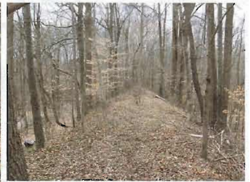
Below: Fill section in Owings, MD. The broad top section and the hill sloping down and away from the trail are giveaways to the trained eye.
